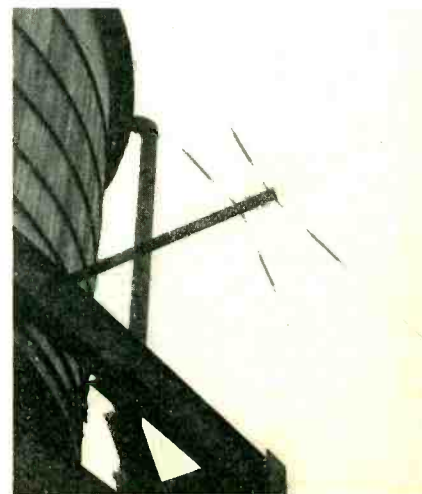
How a water tower on the roof is used as a support for a multi-aerial master antenna system.
